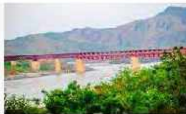
Attock Bridge an Engineering System
