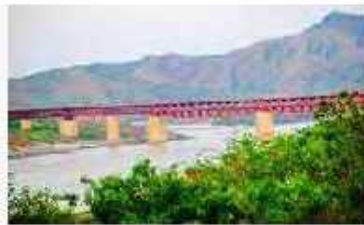
Attock Bridge an Engineering System
