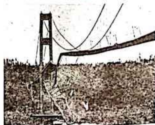
Fig.7.24: After resonance condition Tacoma narrow bridge
