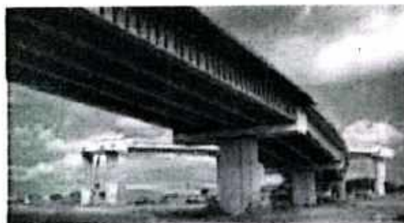
Figure 11.18: Carbon fibre-reinforced concrete.
