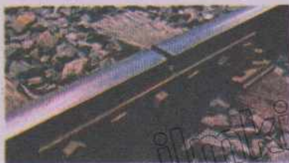
Fig 10.5: (a) Expansion gaps in railway tracks (b) Expansion joints in bridges
