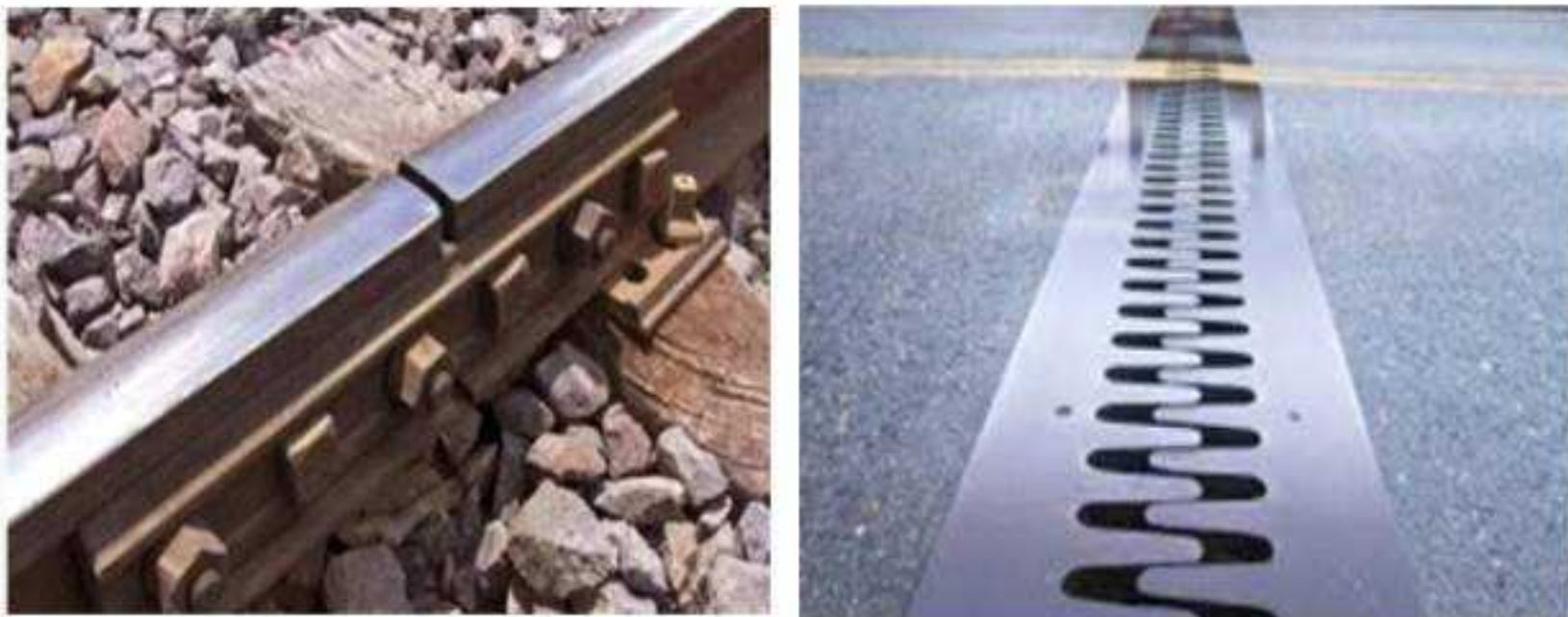
Fig.10.5: (a) Expansion gaps in railway tracks (b) Expansion joints in bridges
