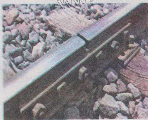
Fig.10.5: (a) Expansion gaps in railway tracks (b) Expansion joints in bridges
