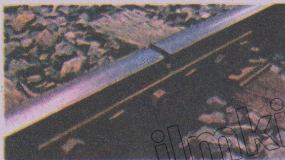
Fig.10.5: (a) Expansion gaps in railway tracks (b) Expansion joints in bridges
