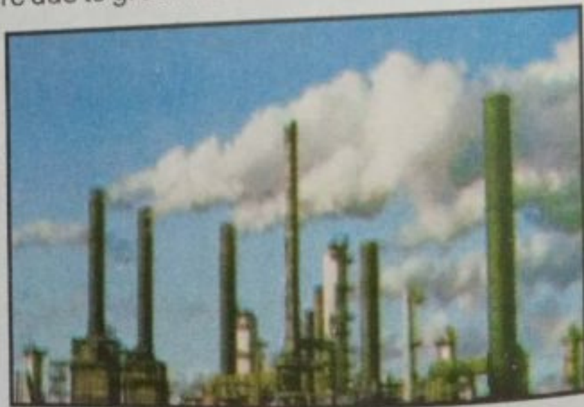
Fig: 5.12 Thermal pollution emitting from chimneys.
