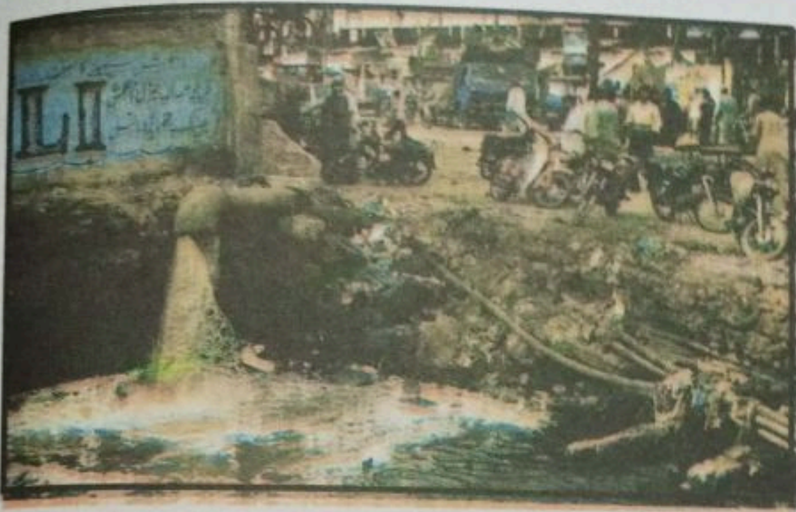
Fig: 4.6 Poor city planning: Easy way for disposal of domestic waste is to open sewerage lines directly into the nearby passing irrigation canals and polluting the precious irrigation water. Rapid trend of urbanization has put tremendous pressure on the old and out dated sanitation system in most of big cities of Pakistan.
