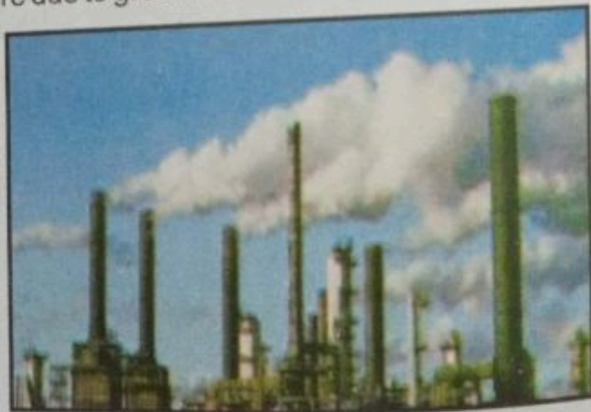
Fig: 5.12 Thermal pollution emitting from chimneys.
