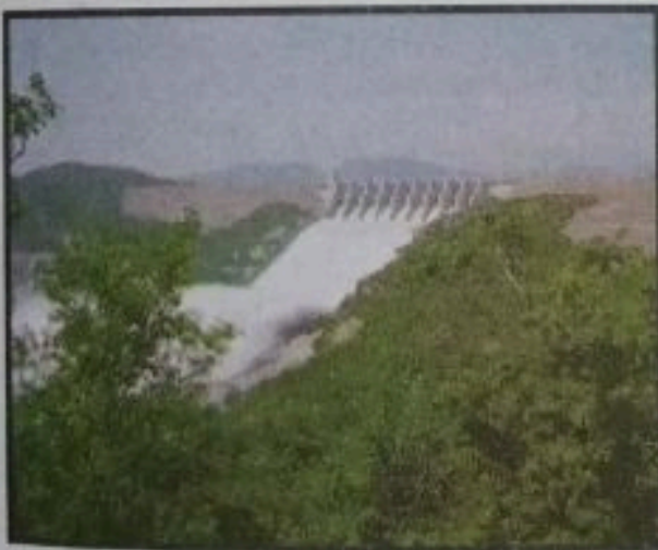
Fig: 4.4 Terhela dam because of which the reservoir has lost the storage capacity to a reasonable level and now the dam is left with two-third capacity to store water.
