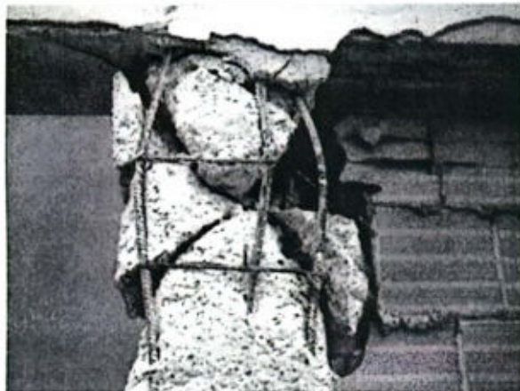
Fig. 10.7: Expansion in construction material
