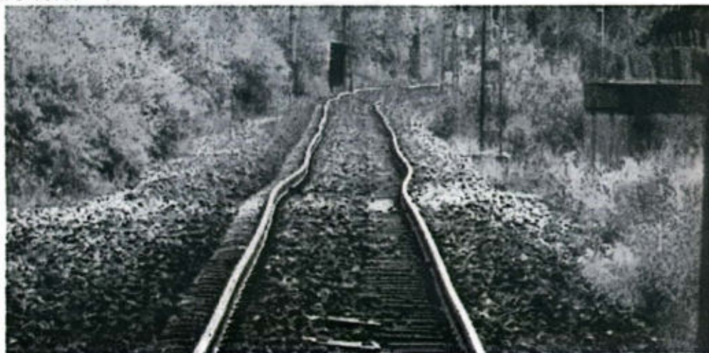
Fig. 10.8: Expansion in railway track
