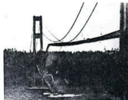
Figure 17.12: Collapse of Tacoma Narrows Bridge in 1940 during a windstorm.
