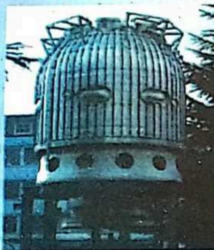
The Big European Bubble Chamber (BEBC) at CERN, near Geneva typical of the large bubble chambers used in the 1970s to study particles produced by high-energy accelerators.
