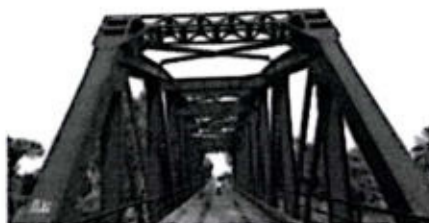
Old steel bridge at Jhang
