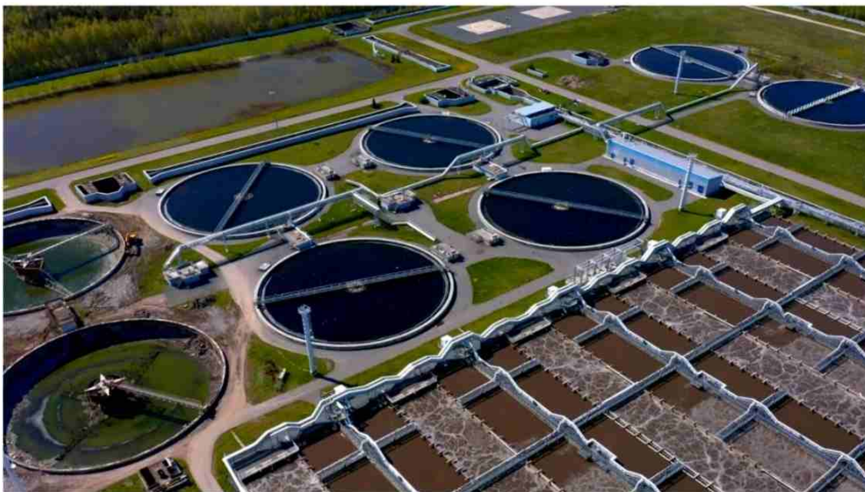
Fig. 27.7 Sewage treatment plant
