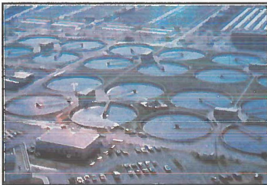
Fig: 27.14 A sewage treatment plant.
